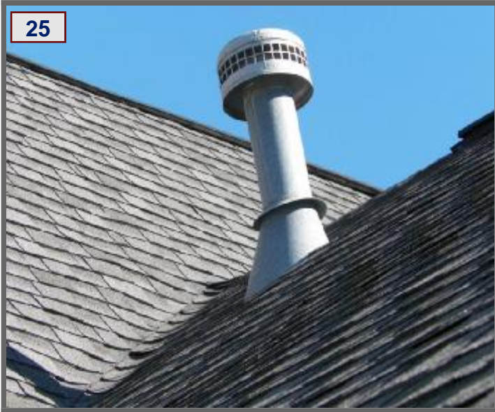
Shingles need secured & sealed at one or more locations.
